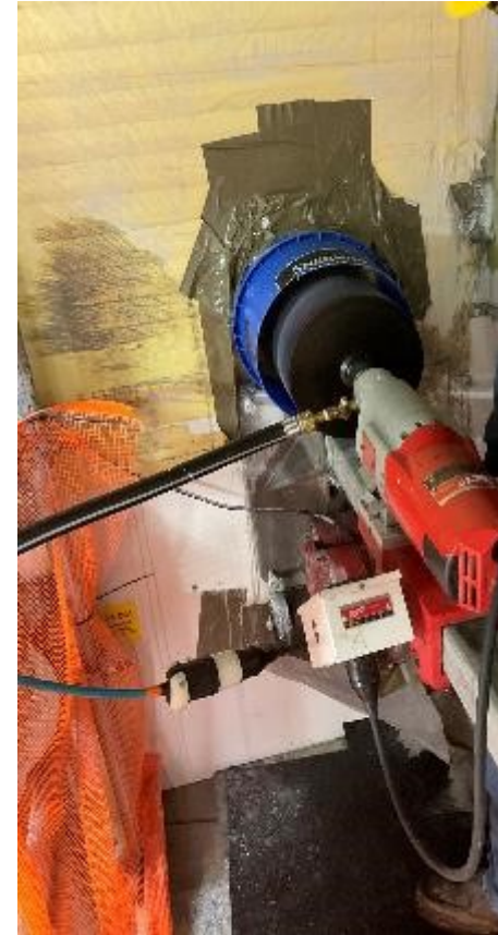
9" Diameter Core Drill for Vibration Monitoring – 36" deep
